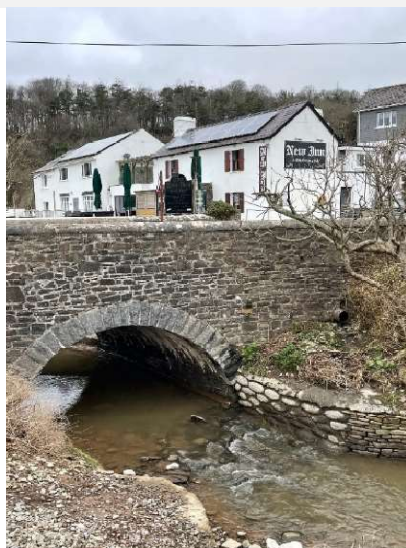
6g. New Inn bridge (Site 8).
