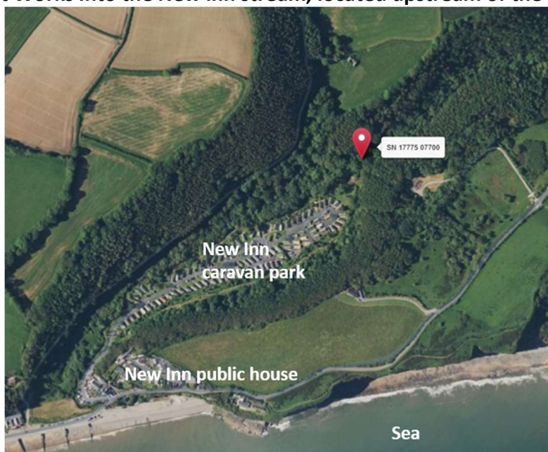
Figure 15a. Location of the waste water discharge (NGR - SN 17775 07700), from the Amroth Wastewater Treatment Works into the New inn stream, located upstream of the New Inn caravan park.
