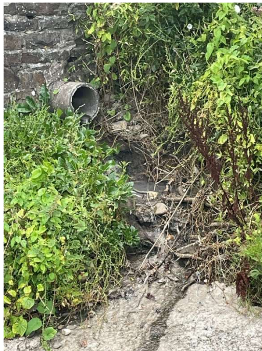
17f) New Inn bridge, 10 th August 2023.
