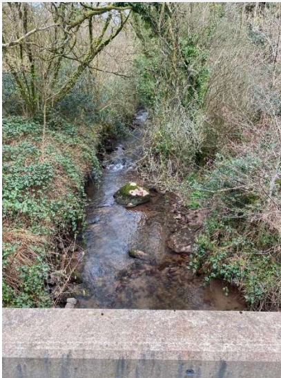
6c. Spiritwood bridge (Site 3).
